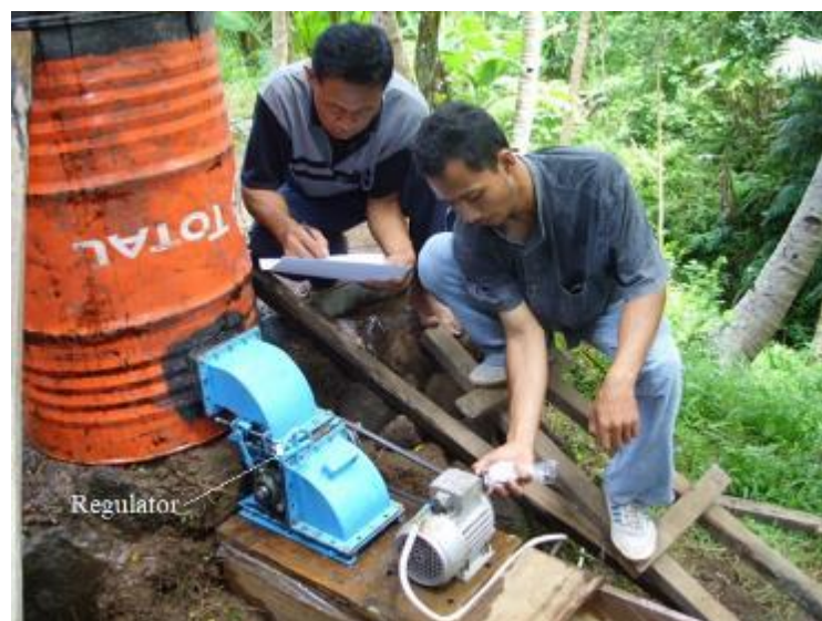
Gambar 10. Pengaturan regulator turbin
